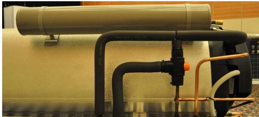
Installation of Pipe Shroud Cover with a HartStat Over Temperature Protection System
